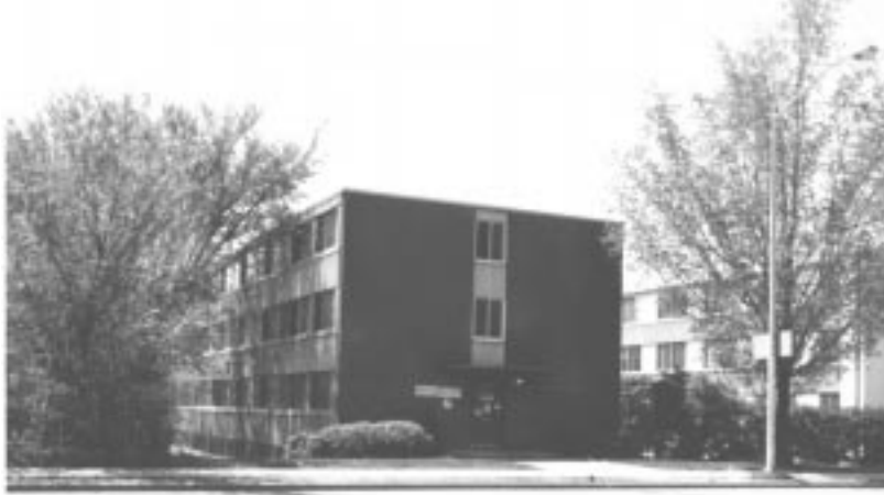
Fig. 1. Zoe Bayliss House 1994: a 32 by 91 foot basement and three floors built of concrete block and poured concrete. Minimal housing for 50 women students. [Author Photo, AP-33]
