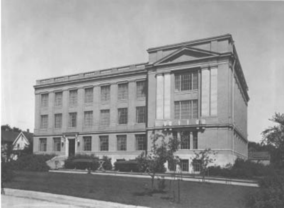
Fig. 1. Wisconsin High School c. 1915. Evident in this photo is the off-center entrance due to a reduction in size from the original plan, without relocating the entrance. [series 9/3, Wisconsin High School, x25-748]
