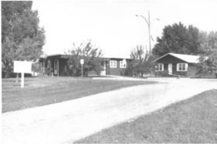
Fig. 1. Day care buildings, 1994. The 1935 flat-roofed building is at left, with the 1965 gabled-roofed one at the right. [Author Photo, AP-22]
