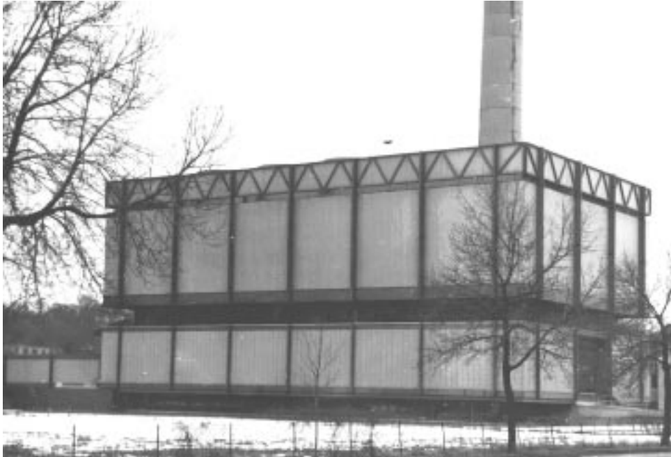
Fig. 1. West Heating plant 1994. [Author Photo, AP-54]
