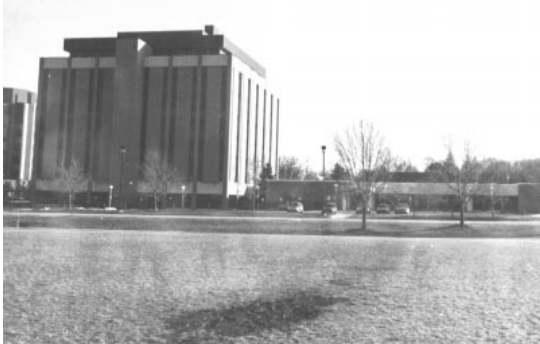
Fig. 1. The Waisman Center, 1995. The school section is at the right. [Author Photo, AP-53]
