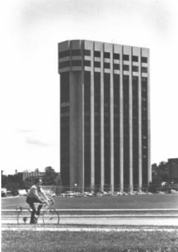
Fig. 1. The WARF building from the north c. 1975. Fourteen stories of concrete and granite, with two triangular floors for WARF at the top. Note how triangular the whole building looks, although only the top two floors are actually triangular in plan. The building will be presented to the University when rents have amortized the costs of erecting the building. [Series 9/3, WARF, jf-91]
