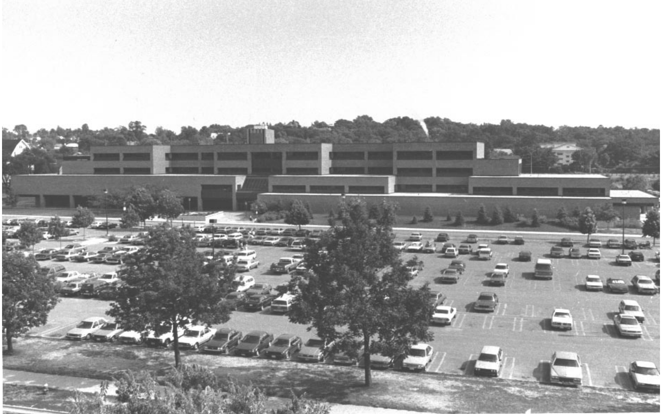
Fig. 1. The veterinary school building, designed by Flad and Associates of Madison, is a four story and partial basement 375 by 225 foot structure of steel and concrete sheathed with face brick and aluminum. The first floor contains the entire teaching hospital and associated services. On the second and third floors are offices, laboratories, classrooms and lecture halls. [photo courtesy of Bernard Easterday ]
