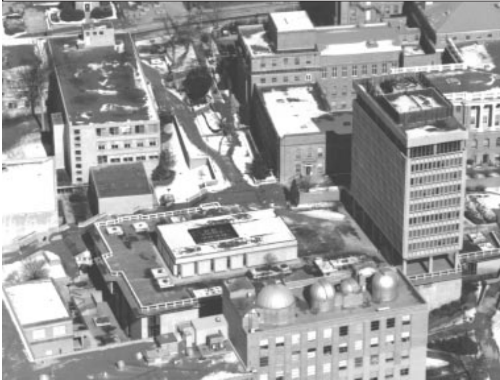
Fig. 1. This photo shows the three story base with roof plaza, the tower section to the east (right). Sterling Hall is in the foreground. Bascom Hall and the Commerce building are in the background. [Del Brown photo, AP-76]
