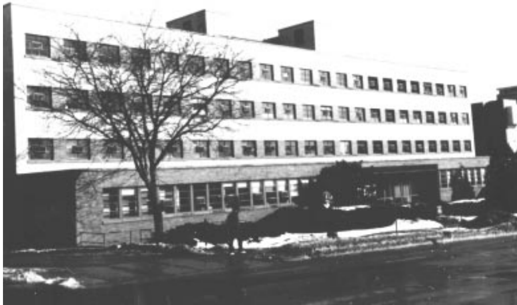
Fig. 1. University Health Services, 1994. The one-story front section could be enlarged to four, and the four story back section to seven if desired. [Author Photo, AP-31]
