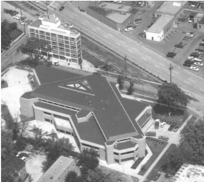
Fig. 2. The odd shape of Union South with its central light well and opening onto a nonexistent court in the back can be seen in this aerial photo. The building is a basement and three levels of concrete faced with concrete and face brick.
