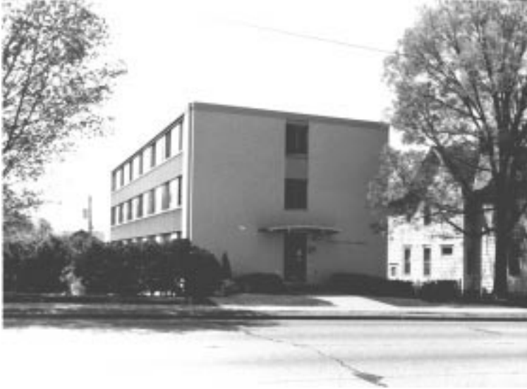
Fig. 1. Davis House 1993. The building is 33 by 91 feet of concrete block, three floors and a basement. [Author Photo, AP-38]
