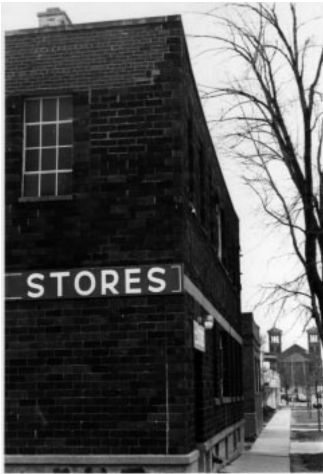
Fig. 2. The old store building at 29 N. Charter Street, 1969. This building was built about 1925 as the Feldman Paper Box Company, and later housed other industrial companies, including Rundle-Spence Plumbing Supply. The University purchased the building in 1958 and moved the University stores operation into it. By the late 1960s the building was deteriorating rapidly. This picture is one of a series taken to illustrate the failing condition of the building. Its foundations had heaved, making the floors uneven, and the basement ceiling was very low because of the installation of modern utilities across the ceilings. Fired danger was considerable because of the storage of flammable gases. A civil engineering professor (John Johnson) was consulted, but his report indicated that the building was too far gone to save. The old stores building was demolished in July 1986 (Memorandum, Kennedy to Fulop, series 4/31/9-3 box 7), after the new Murray Street building opened. The site is now a large parking lot next to the photomedia building.
