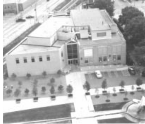
Fig 2. The CAE building from ERB, 1996. Notice the 1987 angled addition (left) to the original rectangular highway lab (right).
