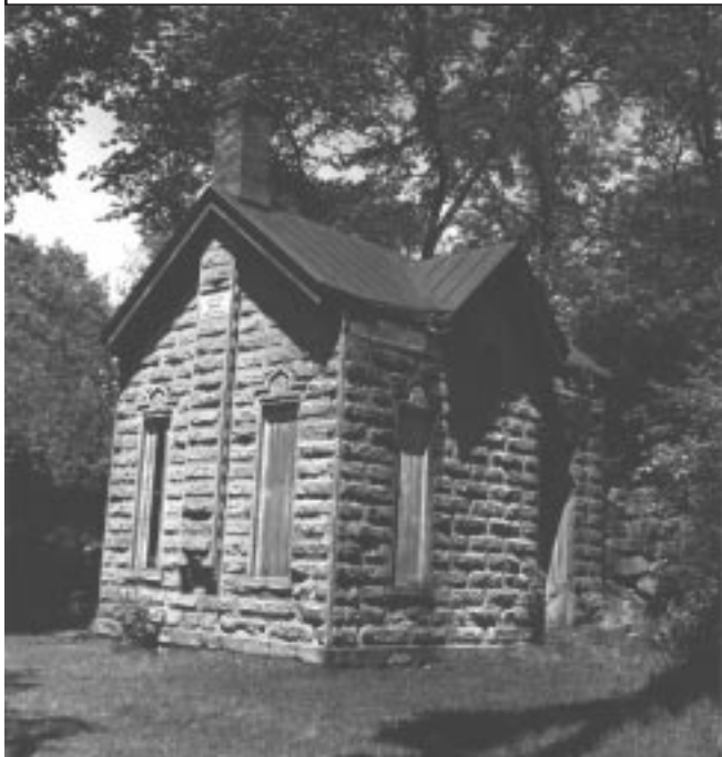
Fig. 1. The Watson Solar Observatory c. 1920. Below the building was a twenty foot deep cellar, and a 55 foot horizontal shaft through the hill to a reflector at the surface on the north side. This building was erected by Professor James C. Watson using his own money and labor. Because of the stone reading "Watson Solar Observatory", the building became known as the Watson Mystery House. [series 9/1 Solar Observatory folder, jf-4]
