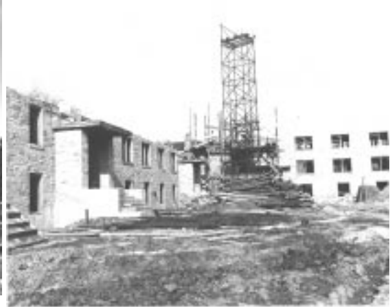
Fig. 2. Construction of short course dorms, April, 1949. [Series 9/3, Short Course Dorms, ns-1724]
