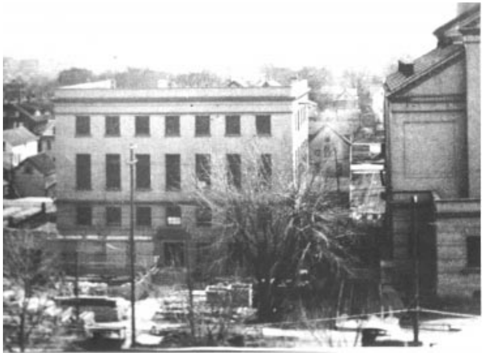
Fig. 2. The original service building, before addition, four stories of concrete with a flat composition roof c. 1910, the central heating plant looms next door. [series 9/5, Heating Plant and Service Building, x25-2924]
