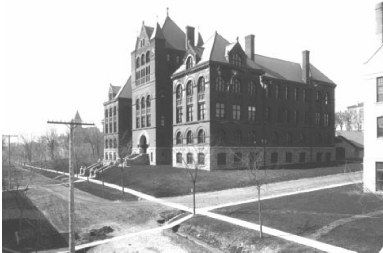
Fig. 1. Science Hall at Observatory Drive and Park Street 1890. Note the board sidewalks that extend clear across the unpaved streets, and the original window in the north wing where a door was later cut. [Series 9/1, Science Hall #1, x25-312]
