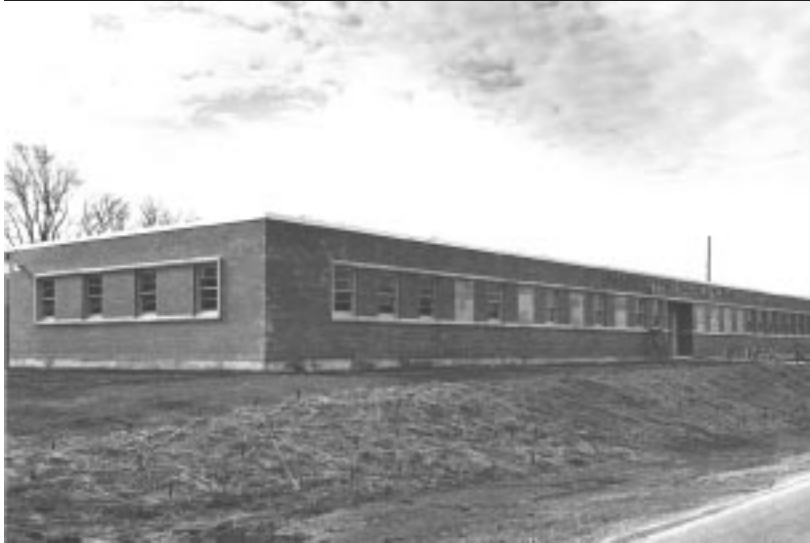
Fig. 1. Poultry Research, just after completion 1957. The building is a one story 43 by 182 foot concrete structure faced with brick. [series 9/3, Poultry Research Lab, ns-2372]
