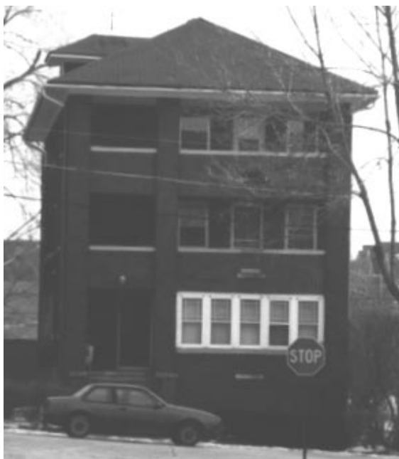
Fig. 2. This 6,912 square foot vintage 1925 apartment building was home to the University Protection and Security department from 1962 to 1989. By the early 1970's it was extremely crowded. The Mills Street facility was about half the size needed, and lacked handicapped access, had makeshift locker and rest-rooms, inadequate storage and ventilation. Parking was very deficient and some records were stored at another old house at 919 Spring Street (since demolished). The women's locker room had no shower facilities. The property and evidence room could only be reached through the men's locker room. After the new building was finished this building was sold, and is now in use as a private apartment building. [Author Photo, AP-59]
