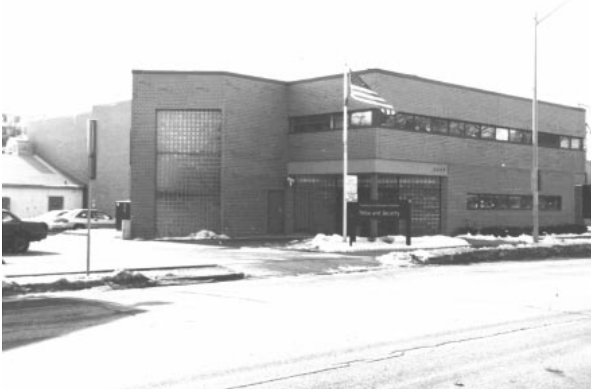
Fig. 1. Police and Security Building, 1995. [Author Photo, AP-58]
