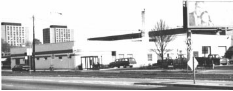
Fig. 1. Physical Plant Garage 1995, a one-story 78 by 52 foot structure of concrete block; the raised section is visible at the right of the picture. The Stores/Extension-Services building is visible in the background, as are the towers of Ogg Hall. [Author Photo, AP-44]
