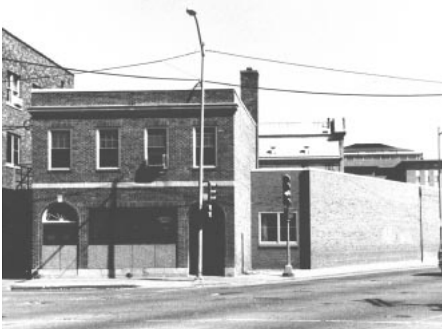
Fig. 1. 317 North Randall St. 1993. The 1966 addition is at the right. The side facing the camera was the entrance to the old post office. The second story of the front section is only 30 feet deep, and does not extend to the back of the building. [Author Photo, AP-16]
