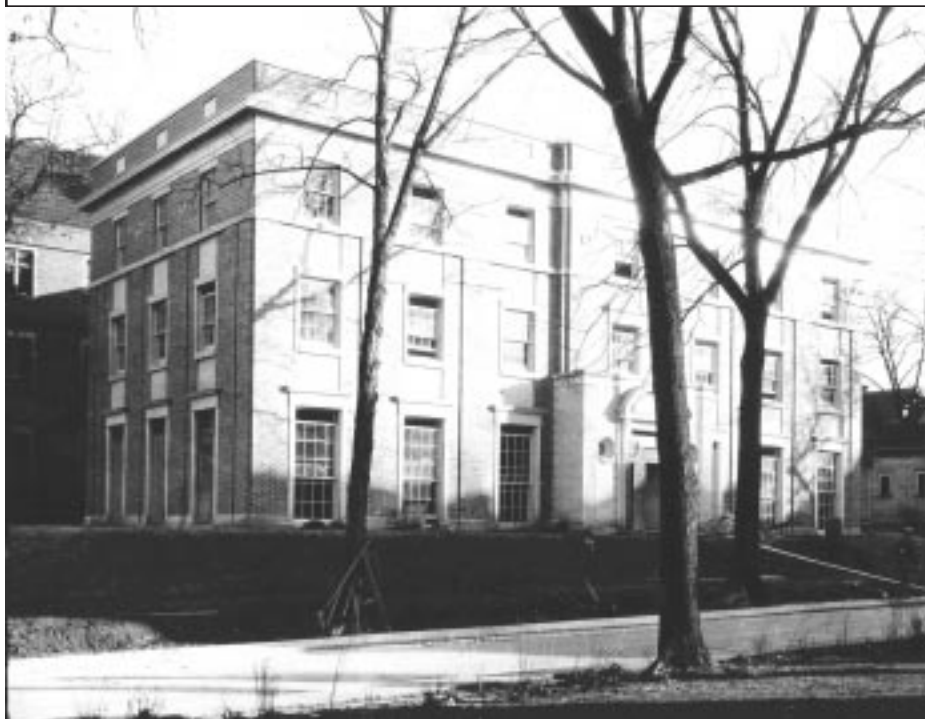
Fig 1. The Phi Kappa Psi house shortly after construction in 1922. [Meuer Photo, vol. 9, p. 48]
