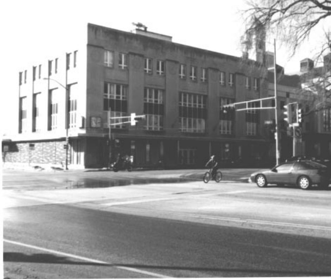
Fig. 1. The old Bank at Park and University Avenue, 1995. 81 by 106 feet, four stories and a full basement built of concrete, with decorative stonework on the street facades. The one story addition faced with lannon stone was added in 1962. [Author Photo, AP-14]
