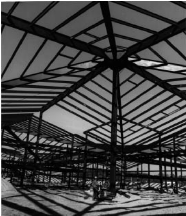
Fig. 2 Construction of the Nielson Tennis stadium, September 20, 1967. [series 7/4 folder #2, jf-100]
