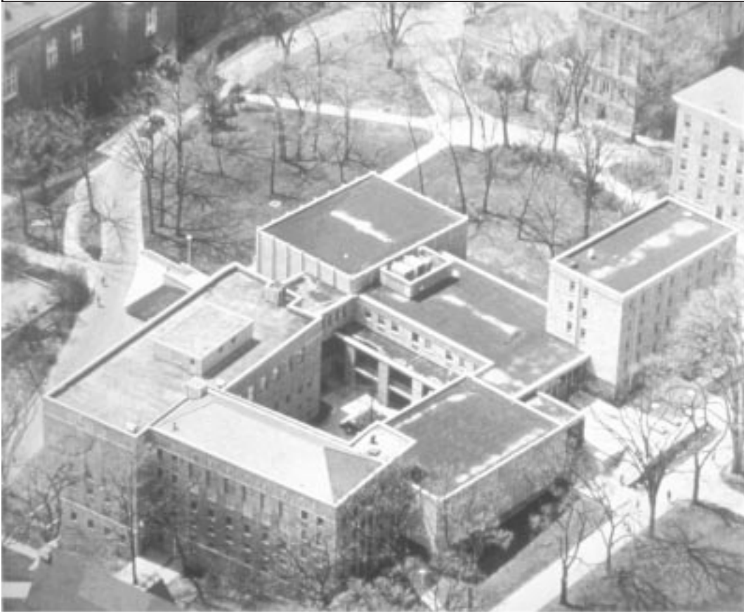
Fig. 1. The law complex c. 1989. The empty area in the center is the location of the original brownstone law building. The 1939 library wing is the L-shaped section in the foreground. The 1959 library addition is the section on the left end of the library. The 1963 construction removed the brownstone, and added
