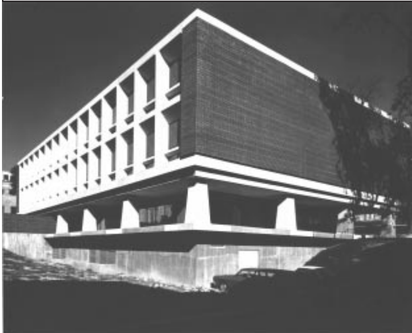
Fig. 1. Middleton Medical Library c. 1970. It is 136 by 82 feet, sheathed in brick on the east and west faces, and concrete panels on the north and south sides, with windows on the north and south sides. [Series 9/4, Middleton Library, jf-85]
