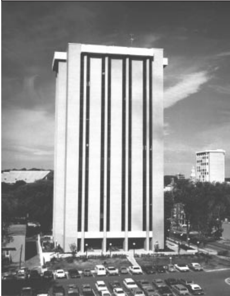
Fig. 1. Meteorology and Space Science building 1972. Fifteen stories of cement block and face brick. Schreiner house at left, Camp Randall and Engineering Research in the far background. In later years the roof of meteorology would become the site of several large satellite dishes, making the building identifiable from miles away. [Series 9/5, Meteorology, jf-87]
