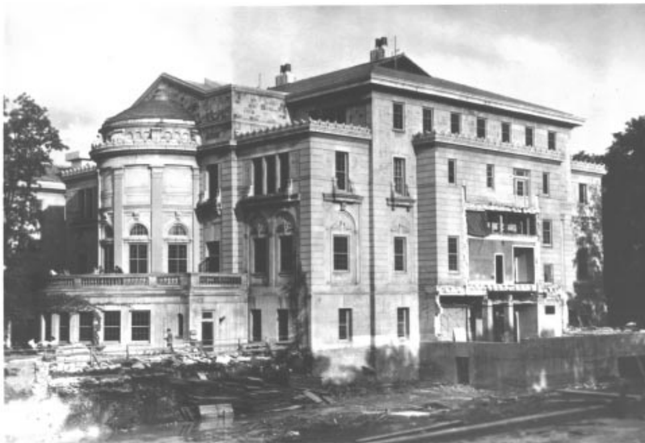
Fig. 3. The beginning of theatre wing construction, 1939. [x25 - 469]
