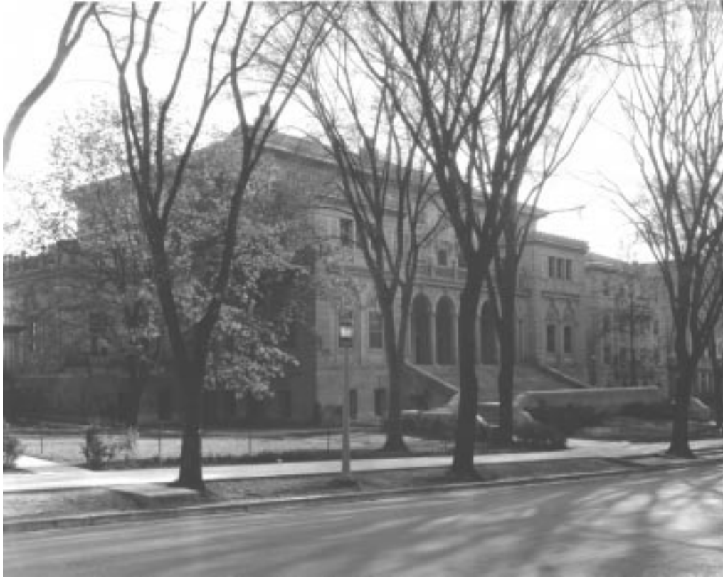
Fig. 1. The Memorial Union from Langdon Street, in 1930. The theatre wing was later built at the left of the picture. Just visible at the extreme right of the picture is the old YMCA, demolished in 1955.
