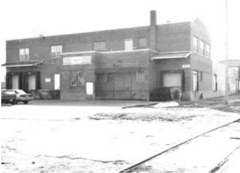
Fig 1. The Medical Supply Warehouse, 1995. The front (Lake Street side) is a basement and two stories of brick, and contains the main loading dock, and office space for ordering and delivery. Behind the front section is a one-story addition that connects to three 40 foot metal quonset sections of one story on a concrete slab. [Author Photo, AP-25]
