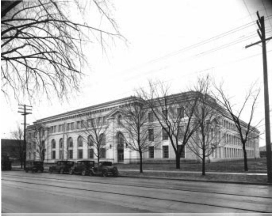
Fig. 1. Mechanical Engineering, 1932. A "U" shaped building of concrete and steel, sheathed with Madison sandstone rubble, some of the last stone to be taken from the west-side quarries. [series 9/6 Mechanical Engineering, x25-586]
