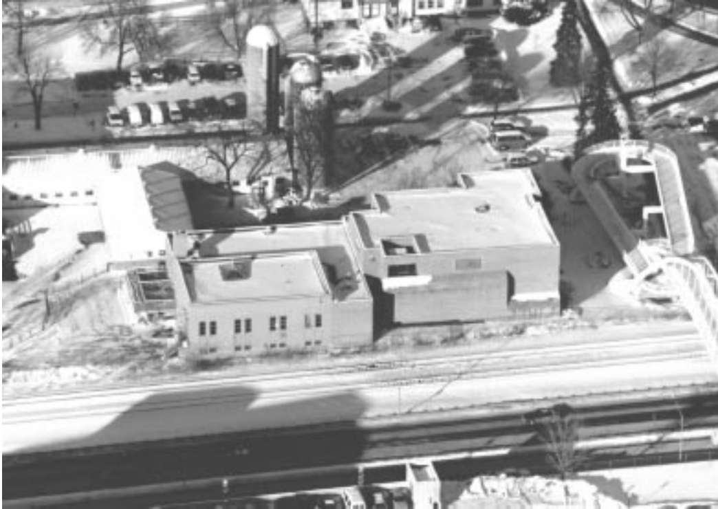
Fig. 1. The Meat Lab February 1997. The original section is at the far left. The 1959 addition is the 'L' shaped section around the original rectangle. The 1969 addition is at the right. The dairy center is in the left background. [Del Brown Photo, AP-67]
