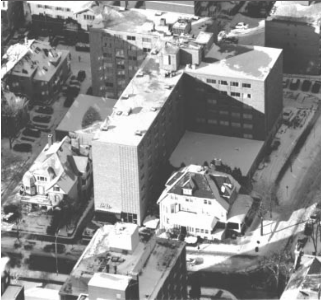
Fig. 1. Lowell Hall February 1997. The stem of the 'T and the right half of the crossbar are the original building. The left crossbar is the 1966 addition. [Del Brown Photo, AP-66]
