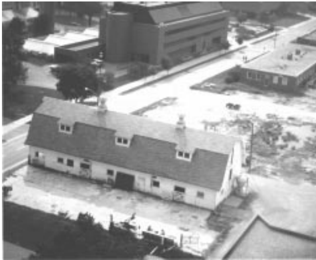
Fig. 2. The old beef barn, just before demolition in August 1991. The beef barn was built in 1924. For decades the departments of meat and animal science were limited to a few old buildings. Besides the old horse and dairy barns (not shown) there were at 1810 Linden Drive two c. 1912 swine barns (already demolished when this picture was taken), and the beef barn. [photo courtesy of Dr. Daniel Schaeffer]
