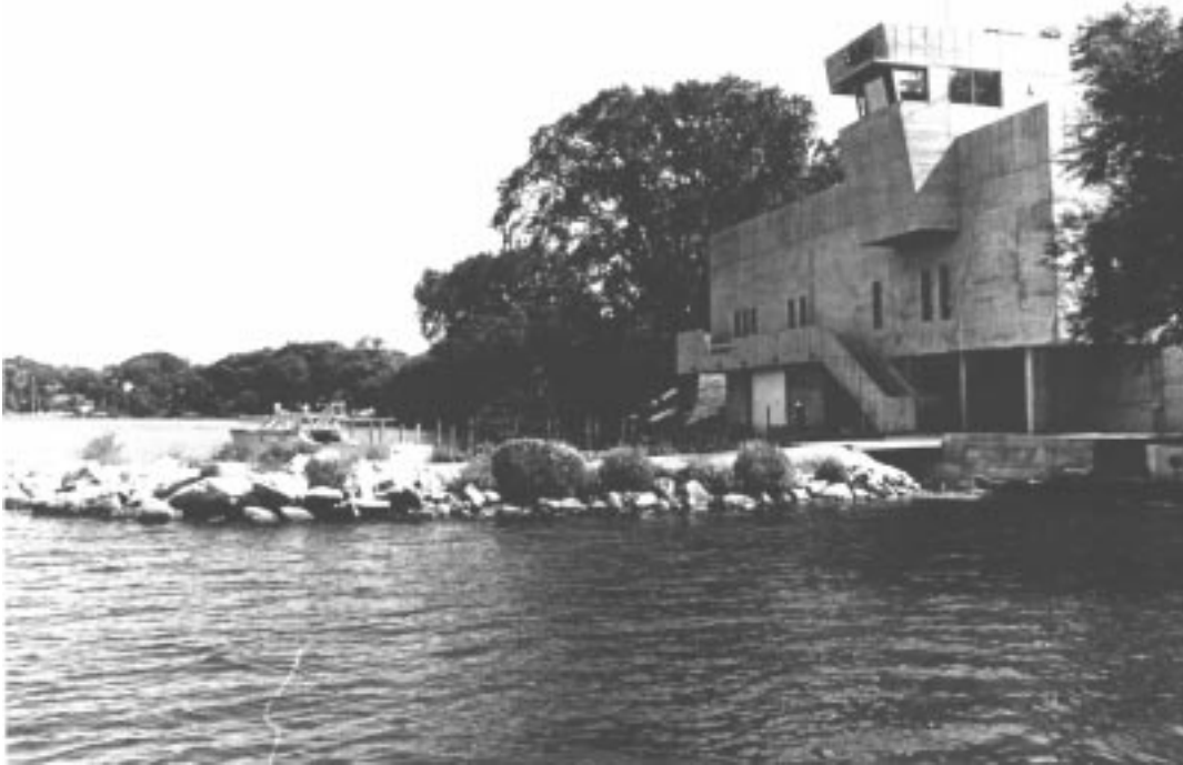
Fig. 1. The Lifesaving Station 1970. The breakwater is at the left; the observation and mechanical decks cantilever towards the lake. [Series 9/2, Lifesaving Station, jf-105]
