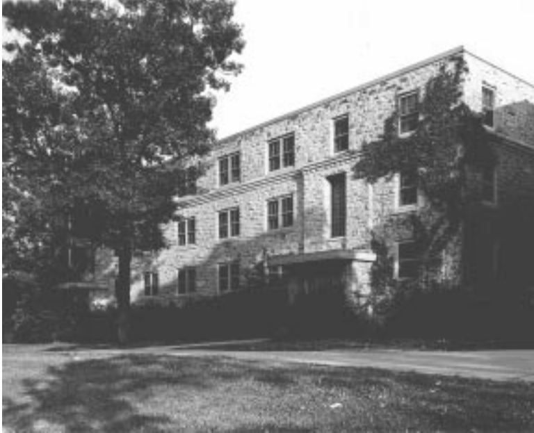
Fig. 1. 1940: Mack House. Mack, Turner and Gilman houses were the first three units of the Kronshage dorms. Three stories with a basement, built of concrete and steel and sheathed with sandstone rubble masonry. They were originally called "A, B and C". [Series 26/1, Kronshage, ns-1519]
