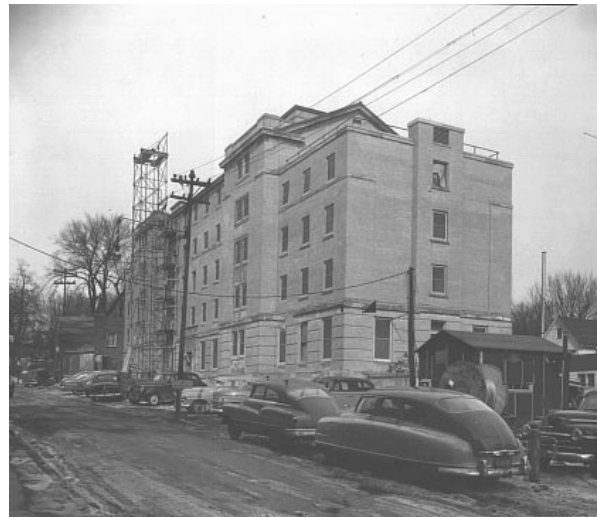
Fig. 3. Construction of the Interns' dorm 1951. [Series 9/4, Intern's Dorm, ns-1502]
