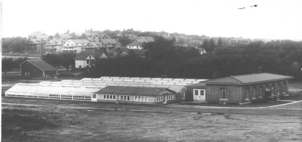
Fig. 1. C. 1911: Horticulture greenhouses from the northeast, farm buildings and the University Heights neighborhood in background. The red-roofed building at the right of the picture is the head house. The little building to the left of the head house is the lab for plant pathology. [Series 9/3, Greenhouses, jf-14]
