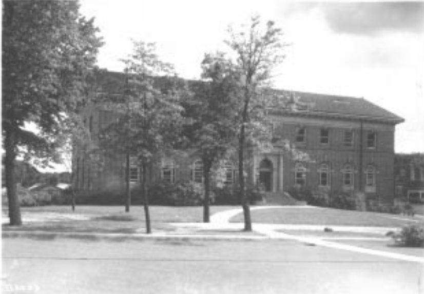
Fig. 1. The original horticulture building from the Linden Street face, c. 1911. [series 9/3 Horticulture, jf-37]
