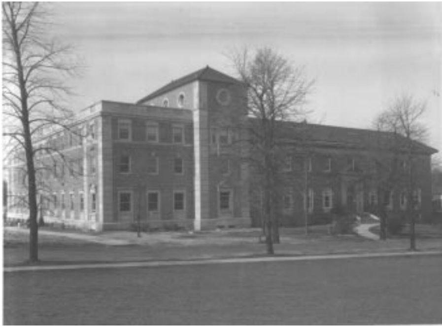
Fig. 2. Horticulture after the addition of the Agronomy wing (Moore Hall), on the left. c. 1932. The tower at the junction of the old building and the addition, disguises the fact that a three story addition had been put on a two story building. [series 9/3 Horticulture, jf-38]
