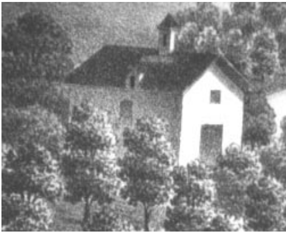
Fig. 2. Detail of 1878 etching, showing original Horse Barn. [etching on wall of Archives] reconstruction of an existing building.
