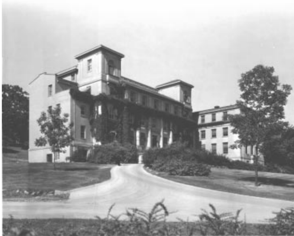
Fig. 1. Home Economics and Extension before construction of west wing; c. 1940. Looking north east. [series 9/3 Home Economics, jf-44]
