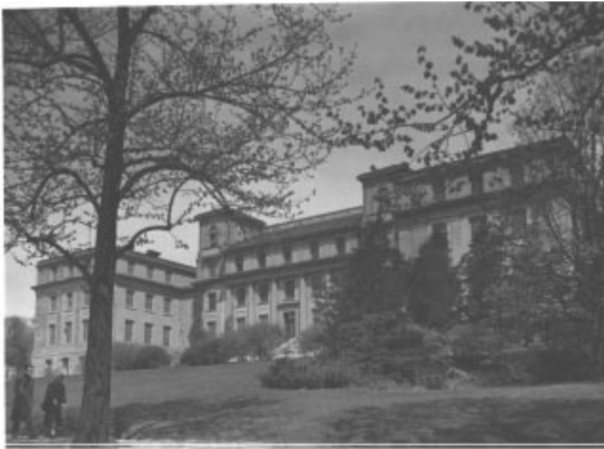
Fig. 2. The Home Economics building c. 1960 after the west wing was built. Looking toward the northwest. [series 9/3 Home Economics, jf-43]
