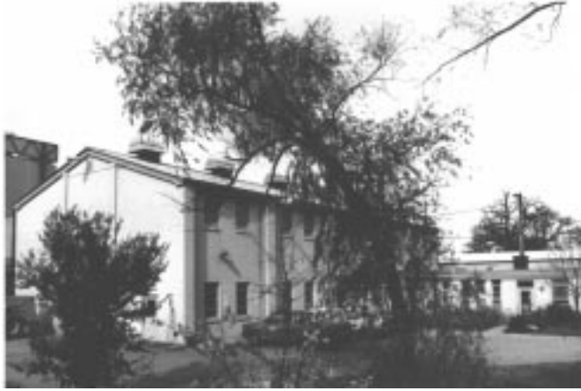
Fig. 1. The High Energy Physics lab in 1994. The building is 'L' shaped, with a 44 by 104 foot shop wing, and a 45 foot one story office wing on the east side. The shop section has a steel frame, while the rest of the building is of concrete block. [Author Photo, AP-39]
