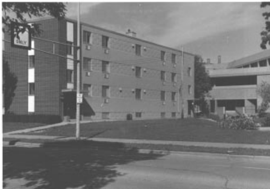
Fig. 1. Hi-Ray Hall from the corner of Orchard and Dayton Streets, 1994. The building is a basement and three stories, 90 by 24 feet. Construction is of concrete block faced with brick, cast concrete and ceramic tiles. [Author Photo, AP-41]
