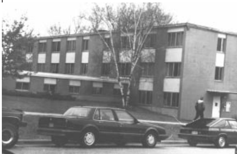
Fig. 1. Rust House, 1995. The central wing is the kitchen addition connecting Rust and Schreiner houses. The building is a 30 by 91 foot three story concrete block housing approximately 55 students in 10 by 12 foot double rooms. [Author Photo, AP-40]
