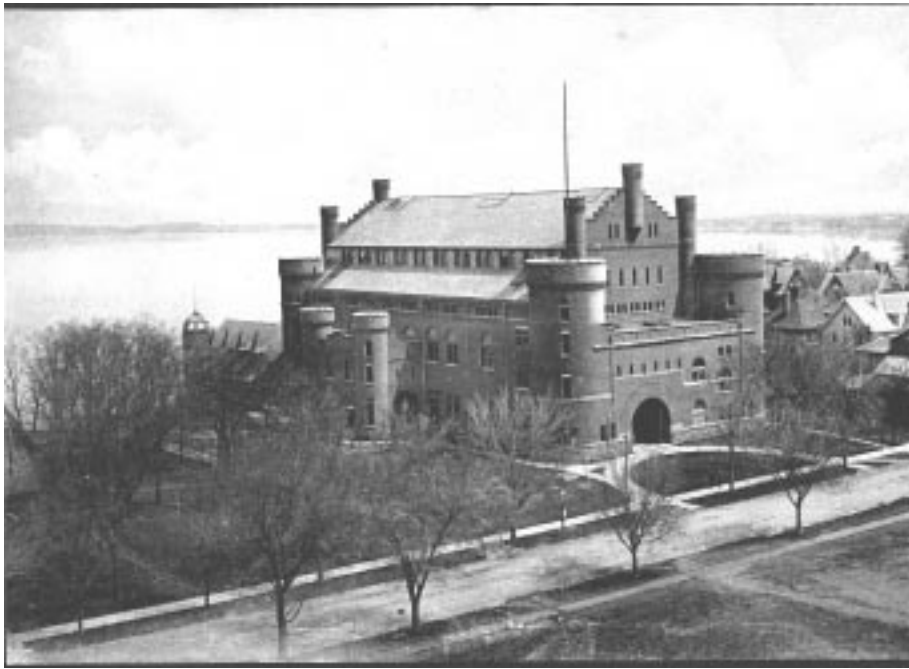
Fig. 3. The gym in its 1899 setting. The houses on the right were removed 1910 for the gym annex and 1956 for the construction of the Wisconsin Center, the old boat house is seen behind the gym at the left. [9/2 armory/gym folder #1 jf-18]
