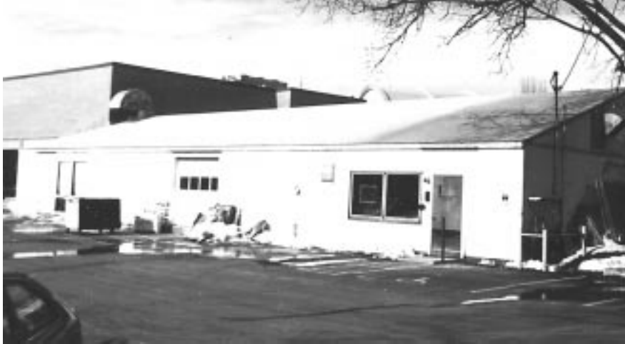
Fig. 1. The glass lab, 1995. The building is a single story, 44 by 92 feet of metal siding over a steel frame with a slab floor. It was probably erected in 1963 by the United Builder's Corporation to be used for lumber storage. [Author Photo, AP-47]
