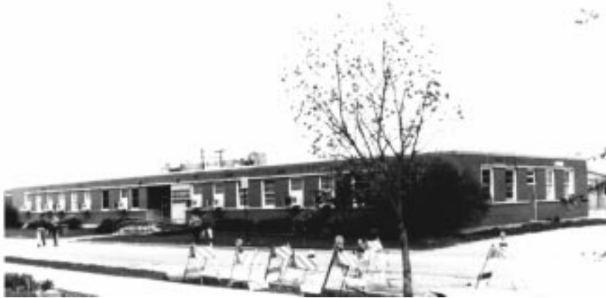
Fig. 1. Genetic research building, 1994, from southeast. It is a 53 by 180 foot one story reinforced concrete building, faced with brick. [Author Photo, AP-37]
