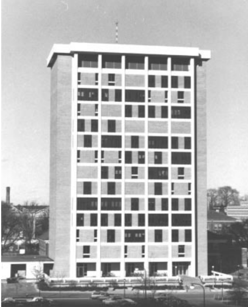
Fig. 1. The Engineering Research Building looking north, c. 1971. The two story base, connected to the mechanical engineering building is at the left. [series 9/6, Engineering Research, jf-90]
