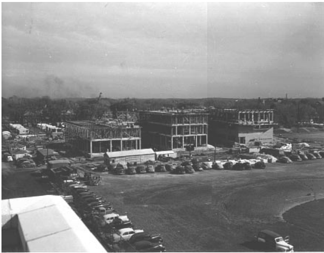
Fig. 2. Construction on west wing October 1949. [Series 9/6, Engineering Bldg, x25-2499]
