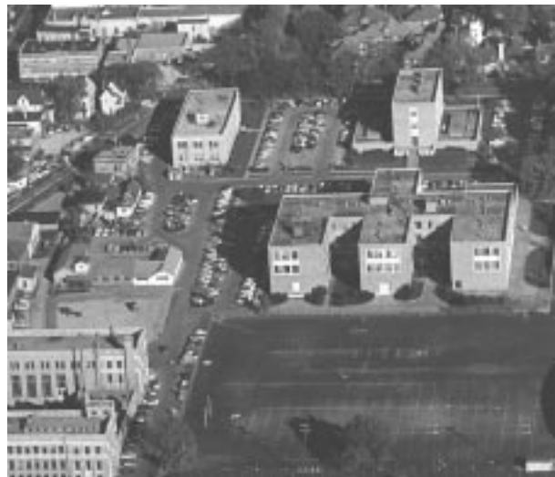
Fig. 3. West wing and chemical engineering section (unit #2) complete, c. 1955. [Series 8/6, jf-64]
