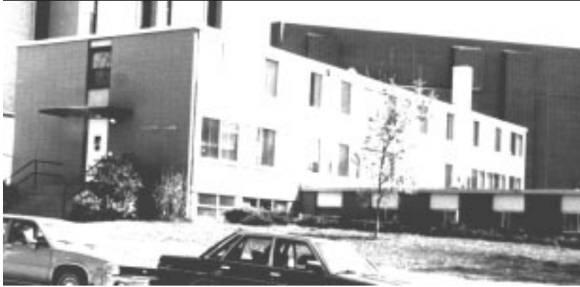
Fig. 1. Schreiner House 1994; a 32 by 91 foot rectangle with basement and two floors of cement block and poured concrete. There were no kitchen or eating facilities. The low structure to the right of the picture is part of the Rust House addition of the 1960s. [Author Photo, AP-34]
