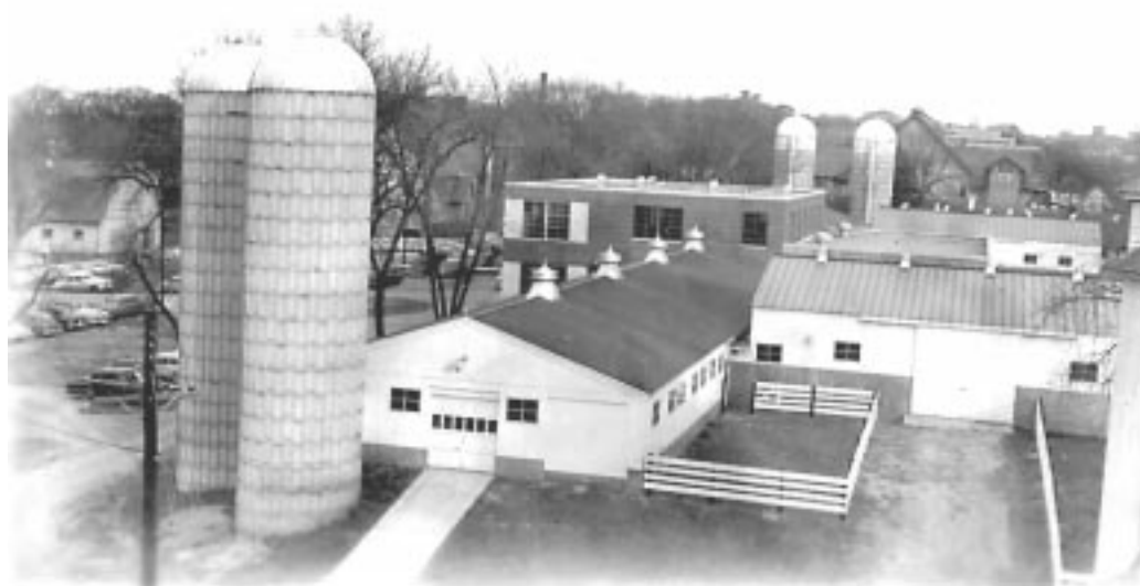
Fig. 1. The Dairy Center November 1954, a two story brick and steel center section 25 by 80 feet, with two 140 foot wings projecting to the east and west. The camera is looking east. The silos in the foreground and background show the extent of the wings. [Series 7/7 folder #1, jf-69]
